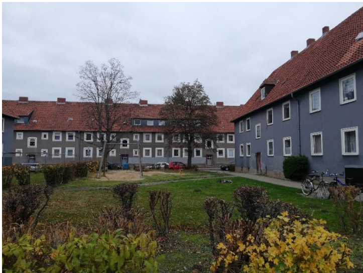
Figure 3: Former housing for migrant workers; Own source
