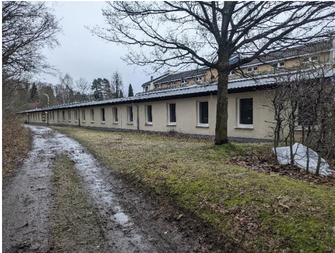
Figure 8: Initial reception center in an outlying district of G-6. Own source.
